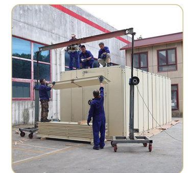
6.Install the roof panel
