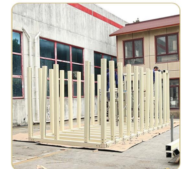
3.Installation of upright posts
