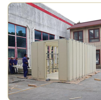
5.Install the side walls
