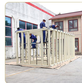
4.Install the top section
